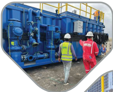
RIG MUD TANK REFURBISHMENT PROJECT
