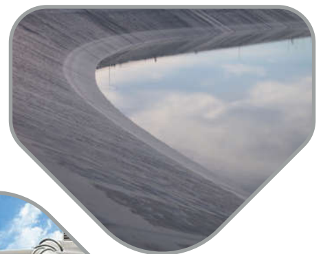
HDPE POND CONSTRUCTION
